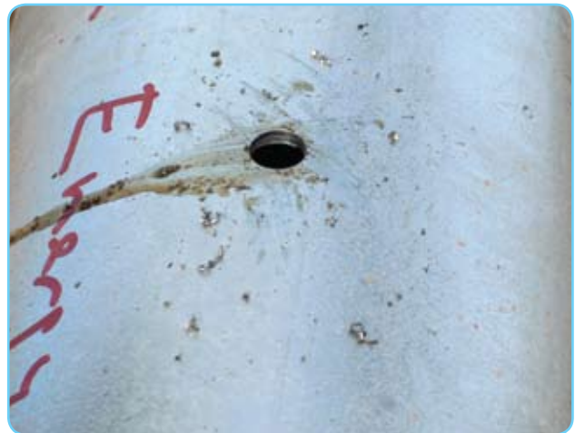
Swarf on pole post drilling
